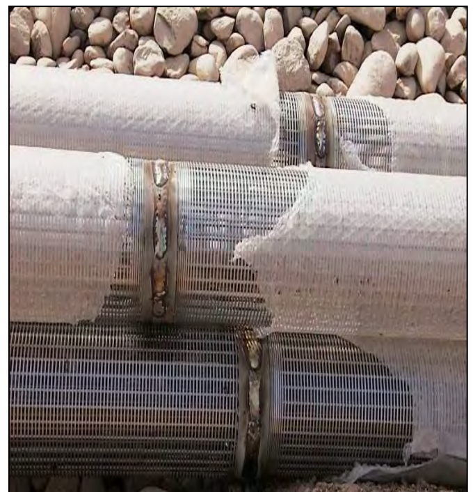
Fig. 9 Picture showing the arrangement and size of the well screens used for the new relief wells at the Karkheh dam
