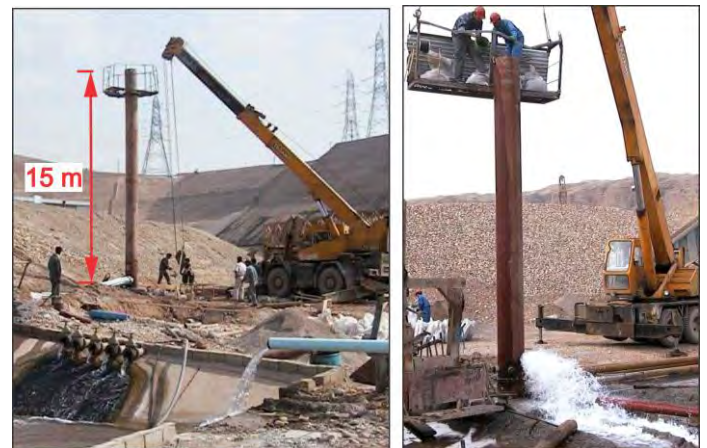
Fig. 5 (Left): controlling the artesian flows by adding long vertical pipes at the top of the relief wells at the Karkheh dam site. (Right): placing filter materials after controlling of the artesian flow
