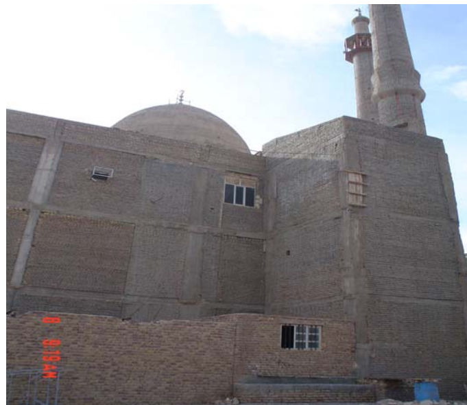
Figure 13. A reinforced concrete mosque after the earthquake which had a satisfactory performance
