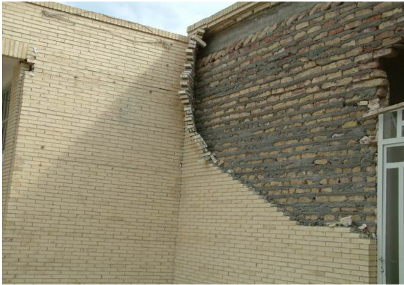
Figure 6. An example of reinforced brick buildings in the earthquake-affected area with a relatively good performance
