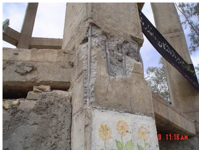
Figure 15. Clos-up view of the cracks in the structural joints of the elevated reinforced concrete water tank tower (note the rebars with no threads).
