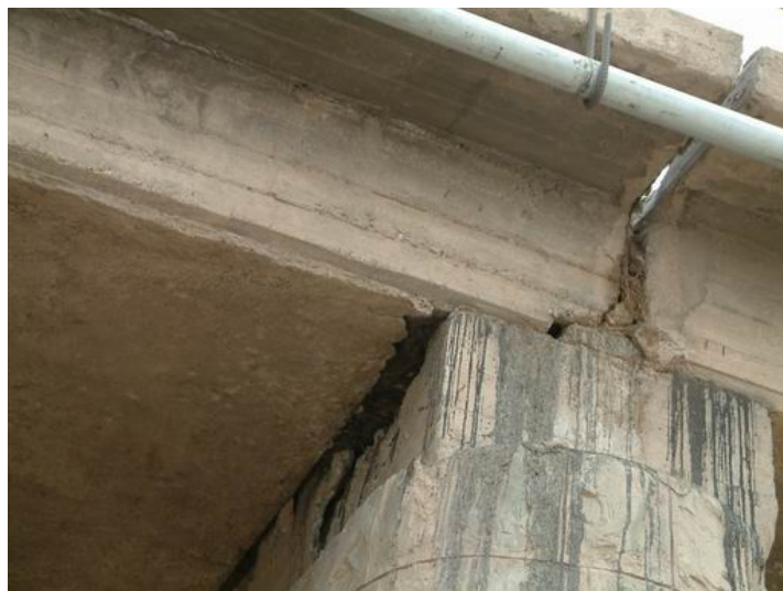
Figure 17. Separation of bridge Spans from the abutment
